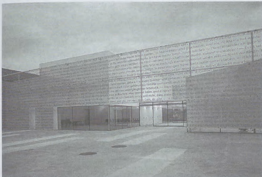
Fot. 5. Centrum Parafialne w Pedersdorf (źródło: < http://www.archello.com/en/project/pedersdorf-parish-centre/image-12 >)
