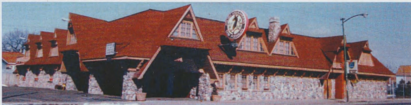
Dom Podhalan – 4808 So. Archer Avenue, Chicago, Illinois
