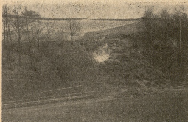
Osuwisko w Kobyle
